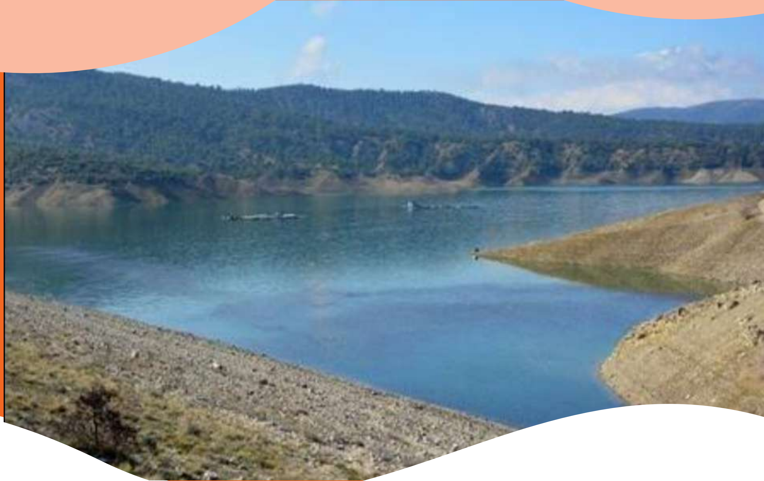
Dam of Korkuteli
